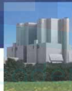
The Schwarze Pumpe power plant (2 x 800 MW), Germany.
